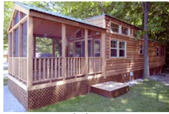
Typical Cabin Exterior
